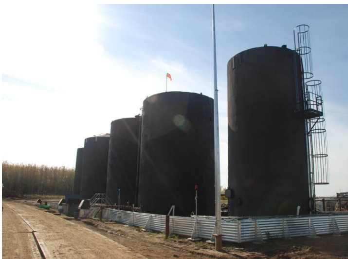
Oil sales tanks at our joint SAGD Project – September 2014.
