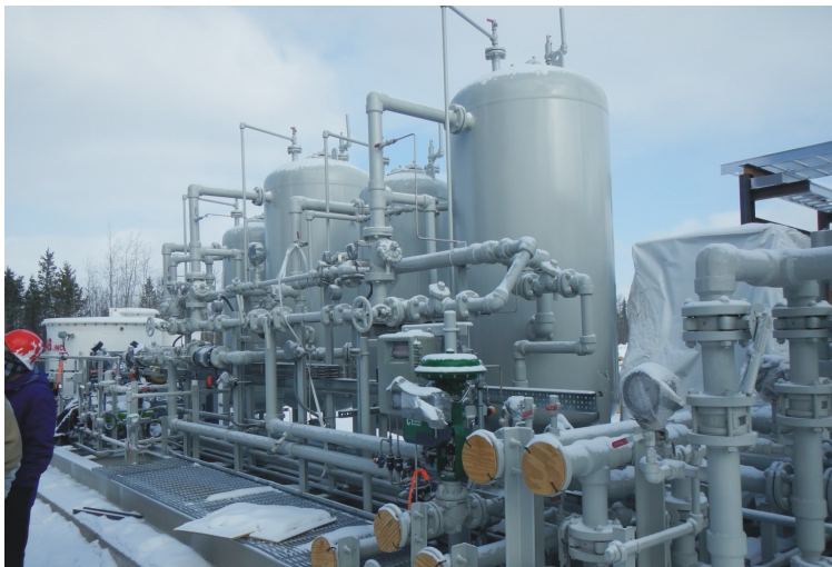
Installation of the water treatment plant at our joint SAGD Project.
